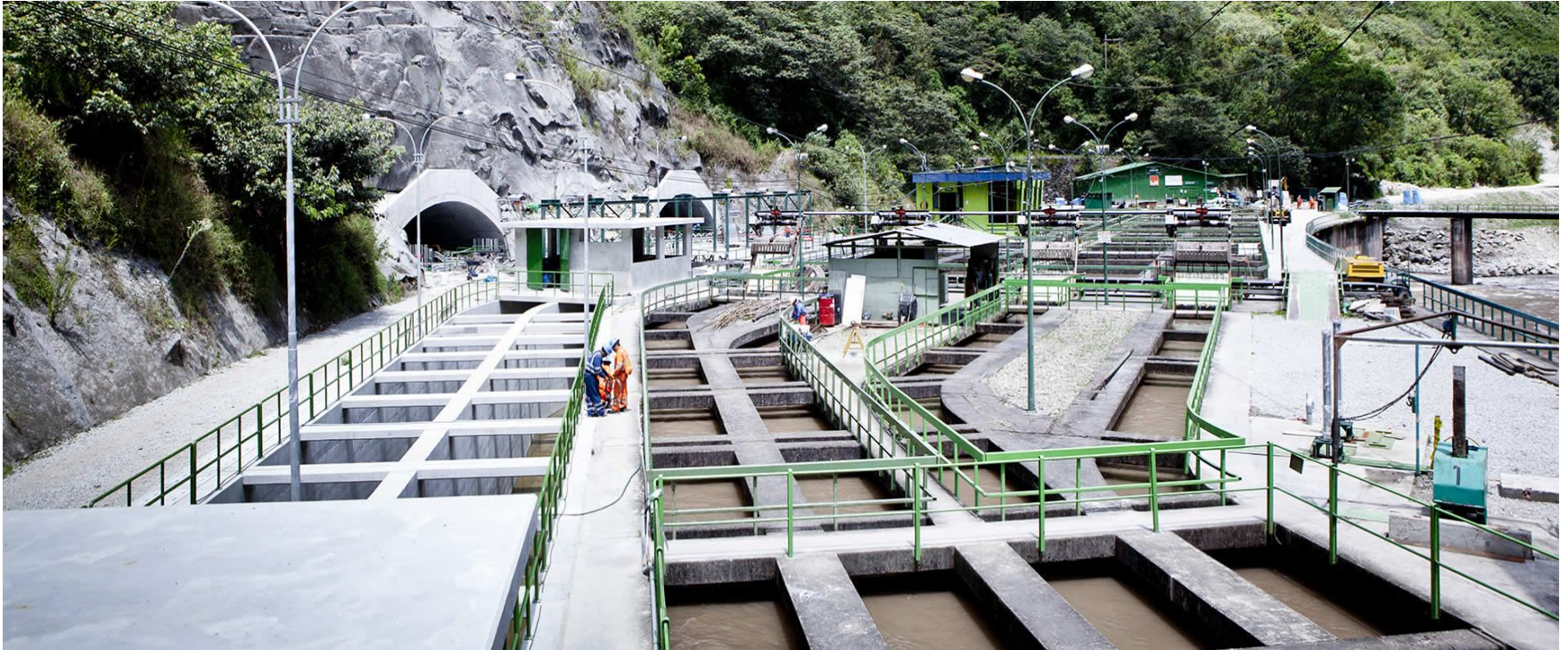
Santa Teresa Hydro Plant in Machu Picchu region
